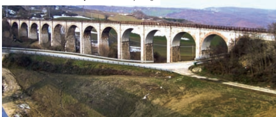
Ponte Ferroviario, Campolieto / Railway Bridge
