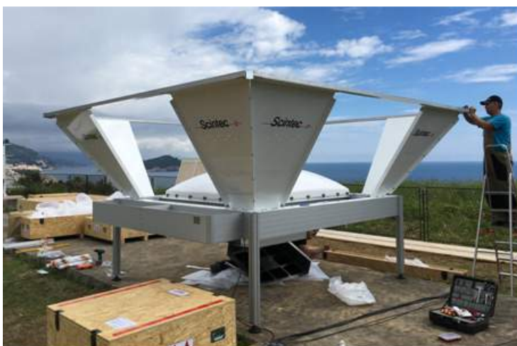
Figure 13 Instalation of wind profiler at GMP Dubrovnik from 21 to 29 May 2019.
