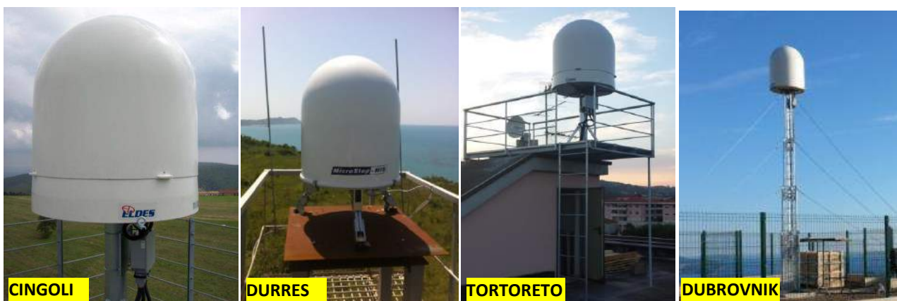
Figure 3.2 Pictures of the four X-band mini-radars installed within the ADRIARadNet project
