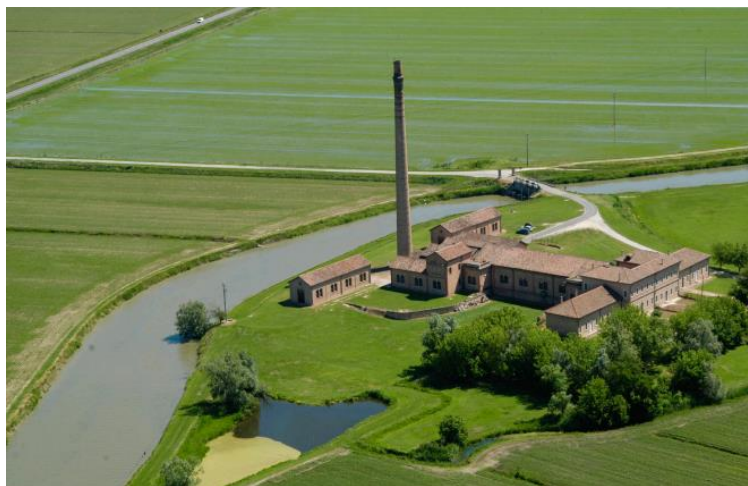
Fig. 1 – Aerial view of the Regional Museum of Land Reclamation Ca' Vendramin, location of the event.
