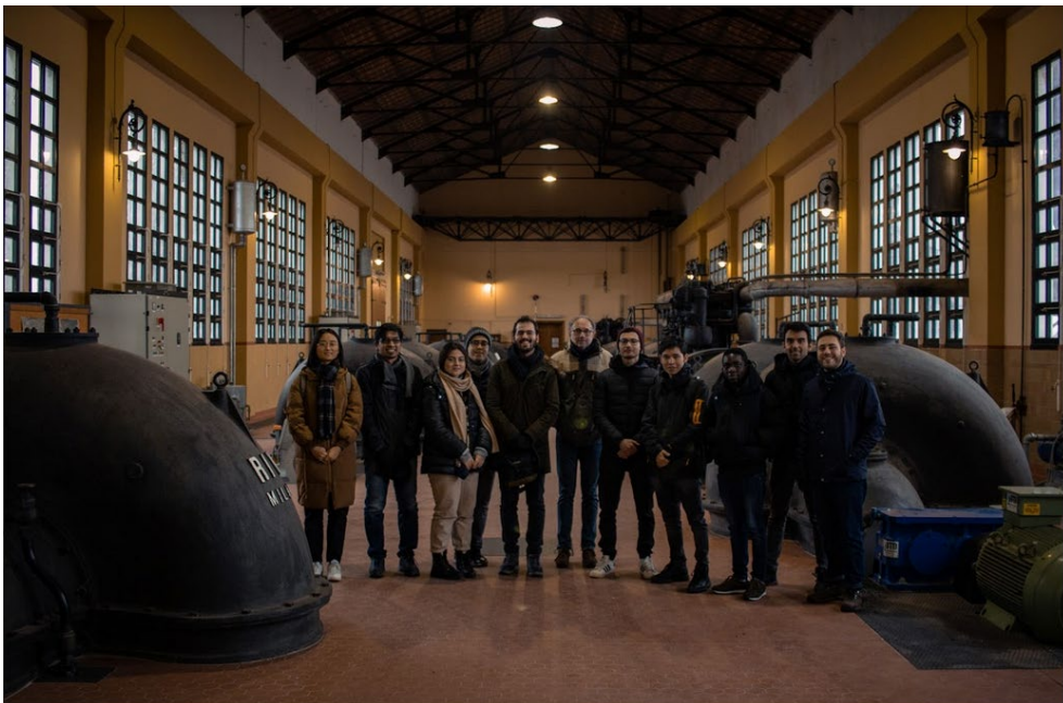
Fig. 14 – December 13, 2022: inside the Ca' Bianca pumping station.
