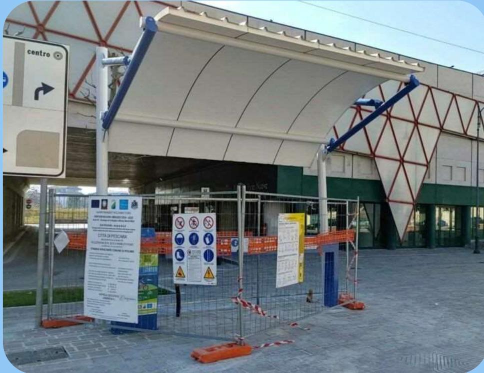
Figure 6.17 – An Eco-Mobility Points under construction (source: Il Pescara local newspaper)
