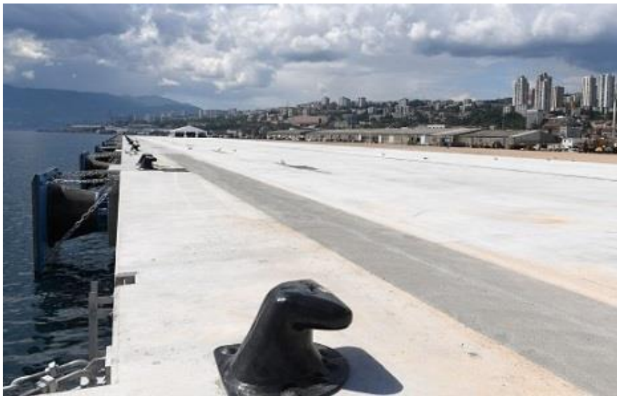
Fig. 4: Zagreb Deep Sea Container Terminal 6
