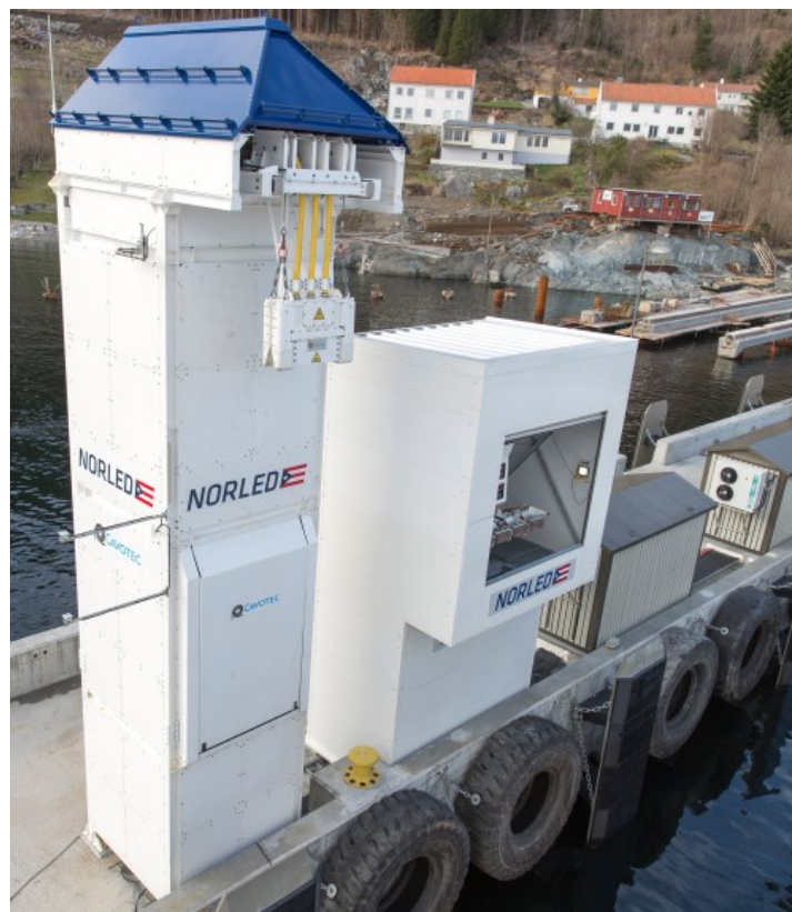
Figure 11. Example of plug in connection for ferries (source: www.siemens.com )
