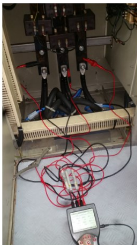
Figure 17. Power measurement on board ferry during voyage between Brestova and Porozina
