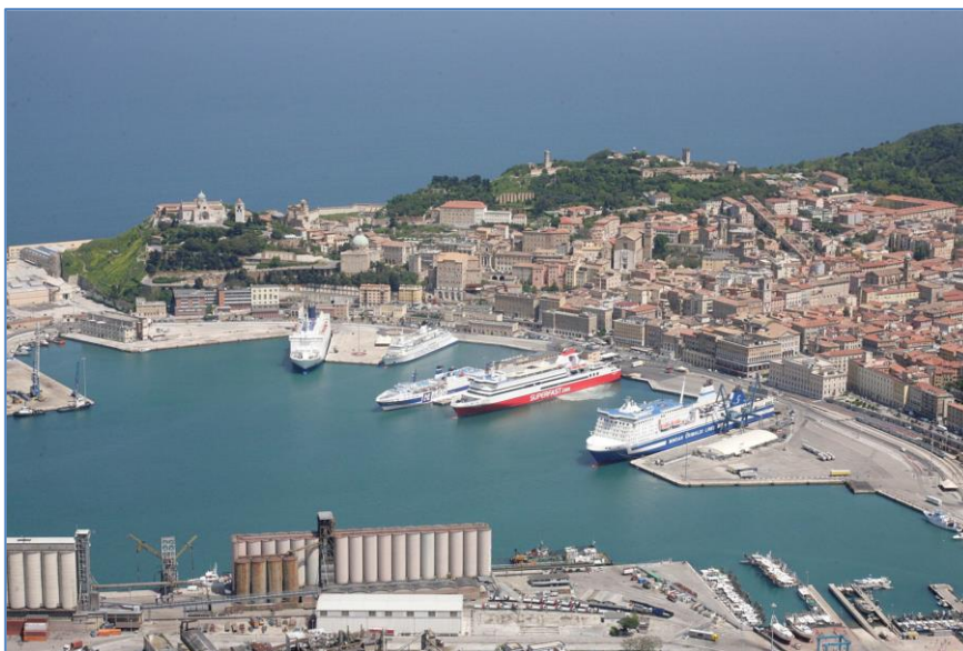
Figure 60 Port of Ancona - passenger terminal
