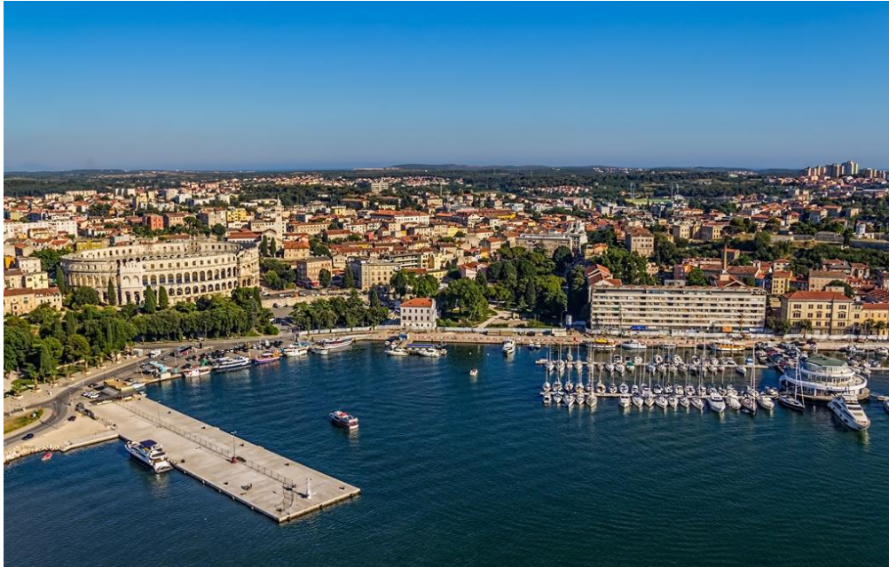
Figura 6: Port of Pula – RO-PAX Quay
