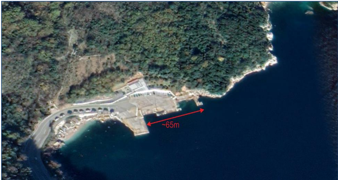
Figure 32 Berth in the port of Brestova
