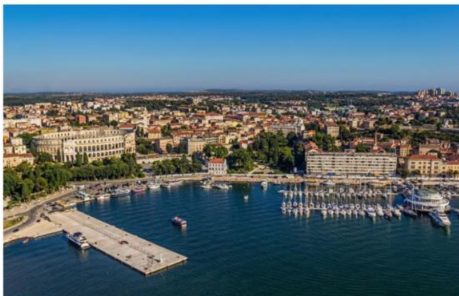
5-17: Port of Pula - RO-PAX Quay
