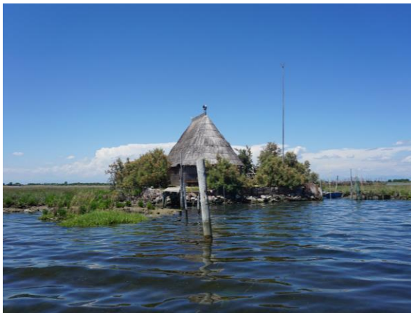
Figure 29. Renovated fishing house
