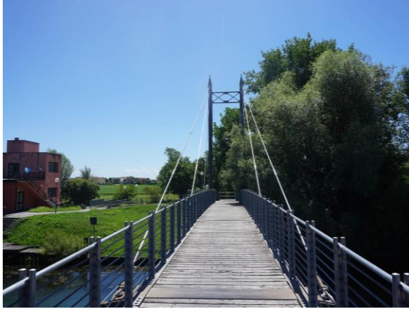
Figure 25. Stella cycle bridge
