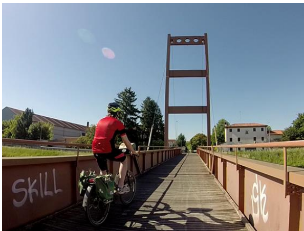
Figure 23. Lemene cycle bridge
