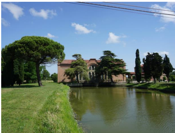
Figure 15. Water pumping station
