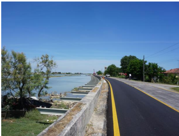
Figure 8. New Pordelio canal cycle path
