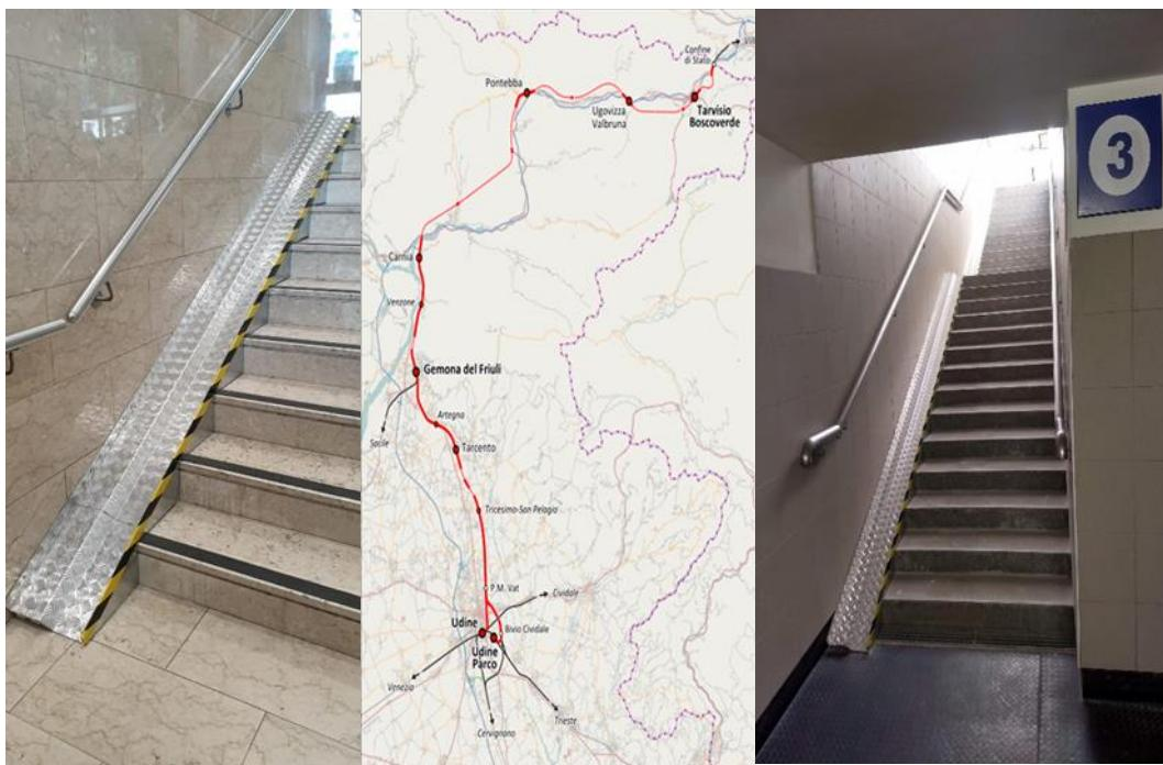
RFI Spa started the works in June 2020 and completed the installation in November 2020. The need for such ramps was underlined by numerous cyclists traveling along the Alpe Adria Cycle Route. This new infrastructure allows all bicycle lovers to access the MICOTRA train (route Trieste-Udine-Villach) and reach the starting points or destination of their itineraries.
