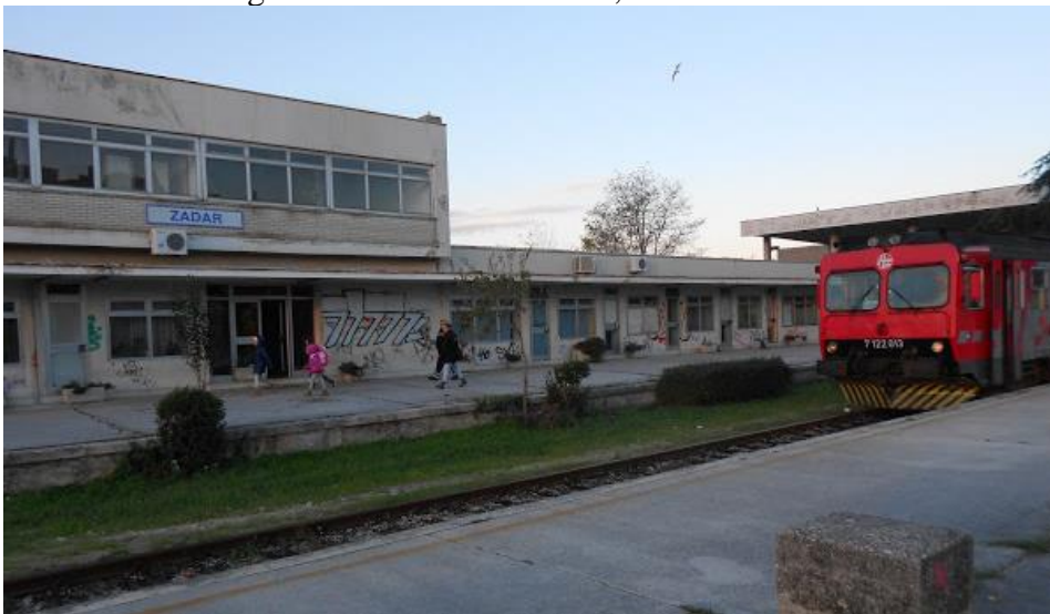
Picture 40: Zadar Railway Station
