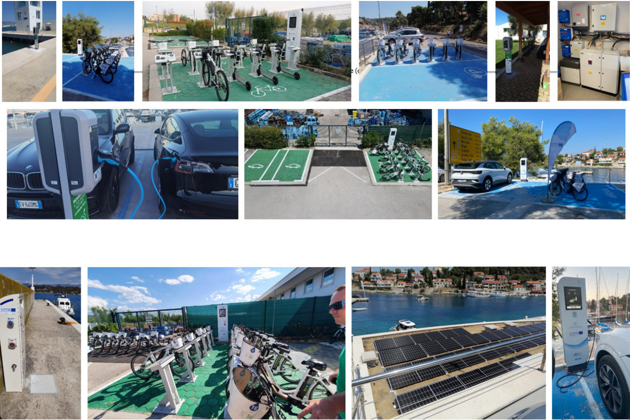
Figure 7 – Installations in DEEP-SEA pilot sites.
