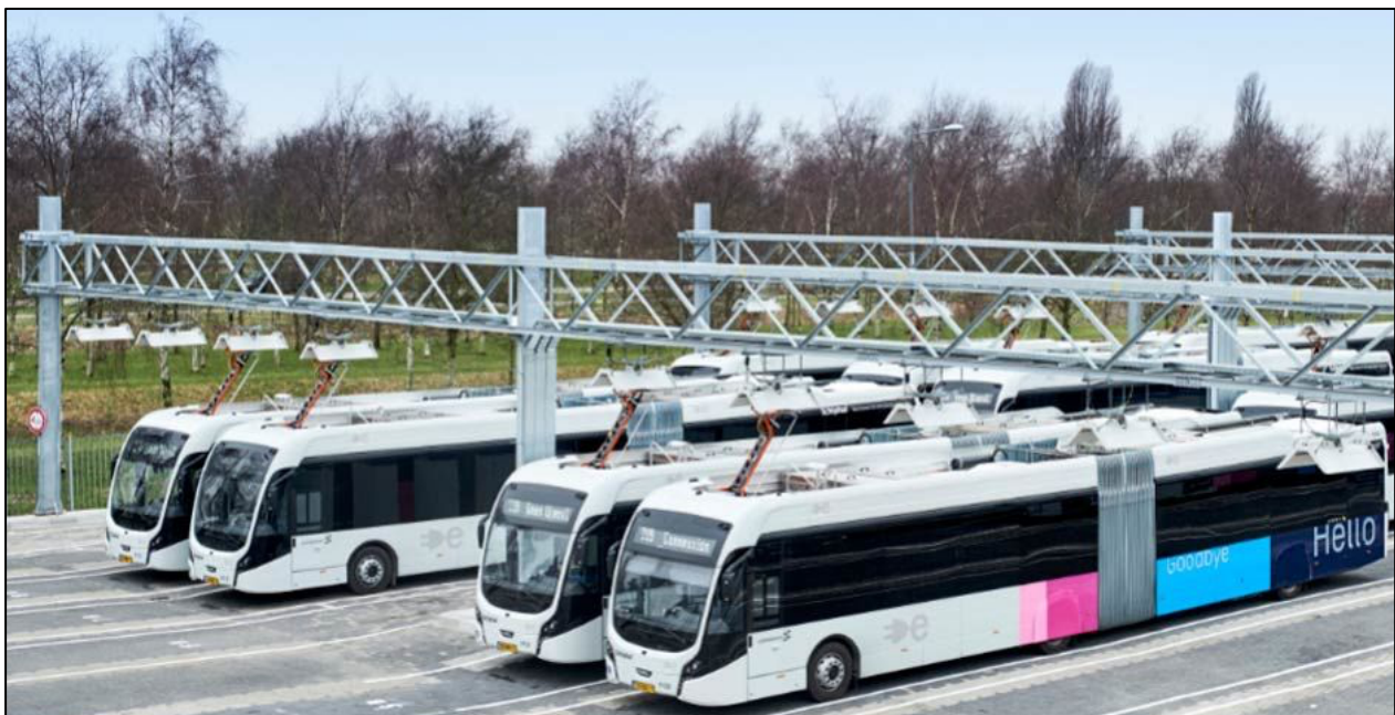
Figure 6. Electric buses at charging station 12 .
