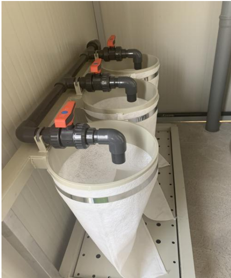
Photographs of the Physical-chemical purifier of wastewater generated during ship washing installed in Marina Strožanac
