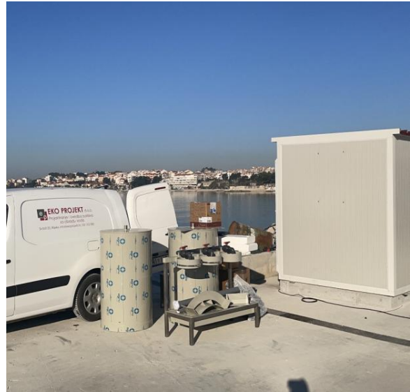
Photographs of the Physical-chemical purifier of wastewater generated during ship washing installed in Marina Strožanac
