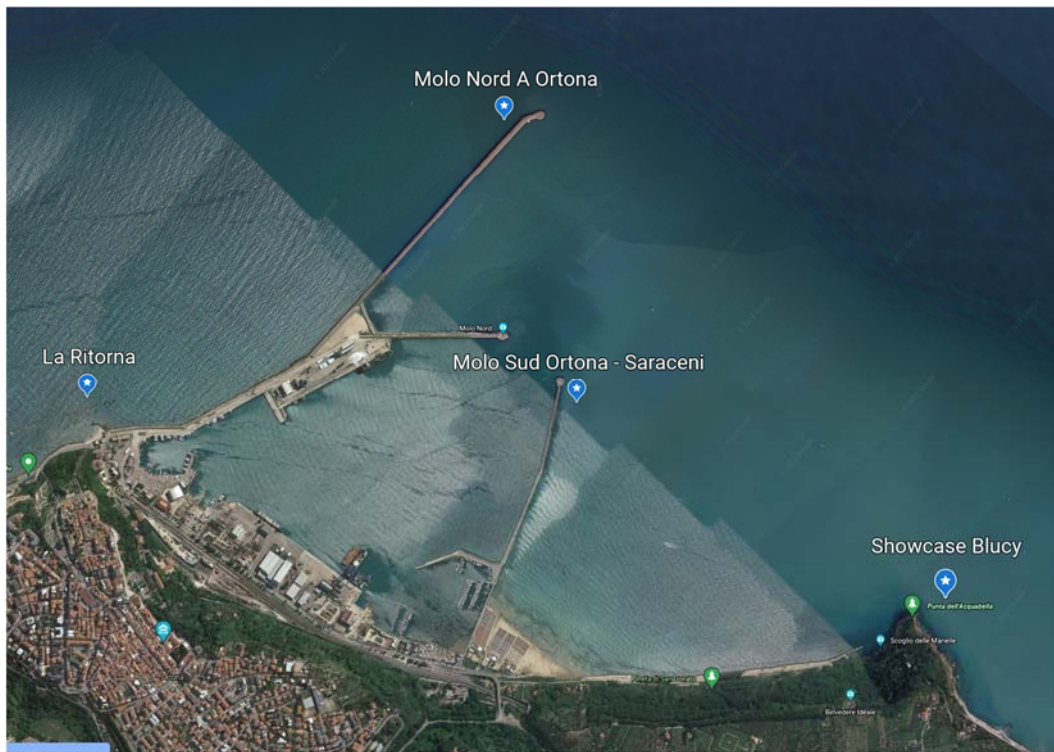
FIGURE 5 MISSIONI SITE IN ORTONA
