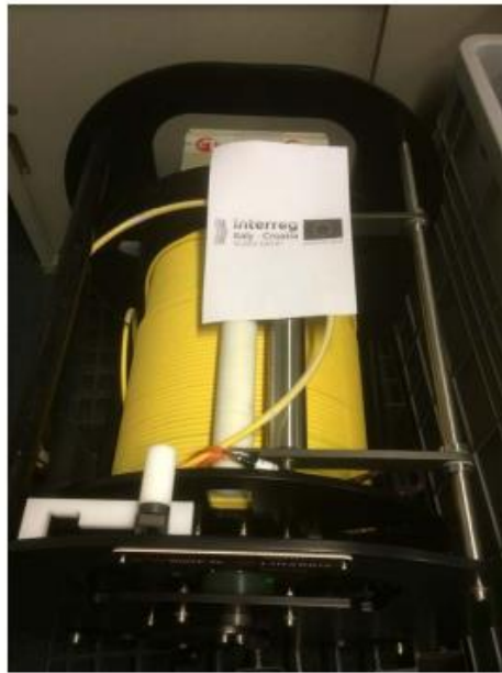
Figure 5 Fyber optic cable + winch
