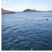
Installation of an environmentally friendly anchoring systems
