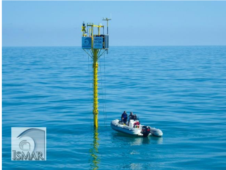
Photo of S1-GB meteo-dynamic pylon
