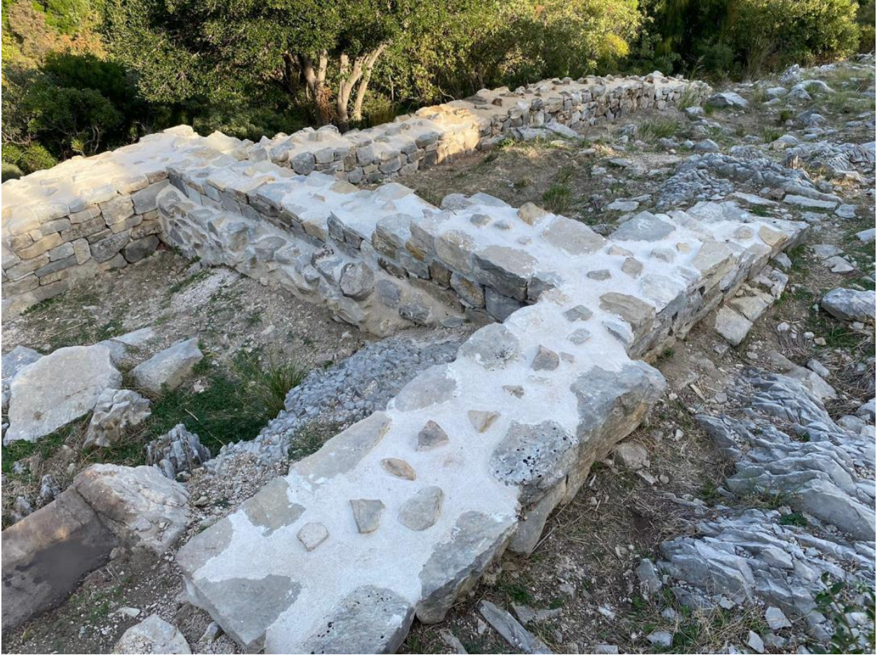
Picture 5. Wall after reconstruction
