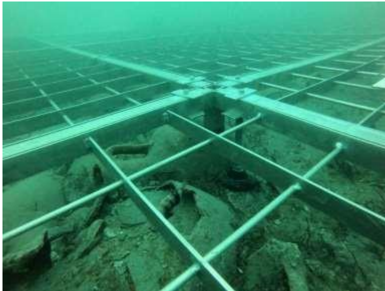
Fig.19: Grado 2 wreck. The underwater grids for covering, protecting and ensuring accessibility to the site
