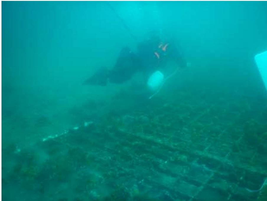
Fig.2 – The removal of the grid
