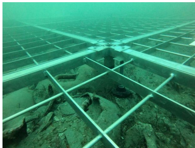
Fig. 3: Grado 2 wreck. The underwater grids for covering, protecting and ensuring accessibility to the site
