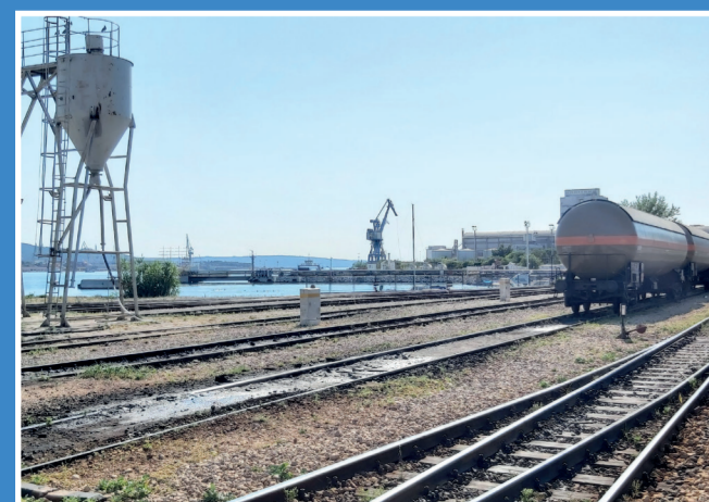
INA tanker berth with crane
