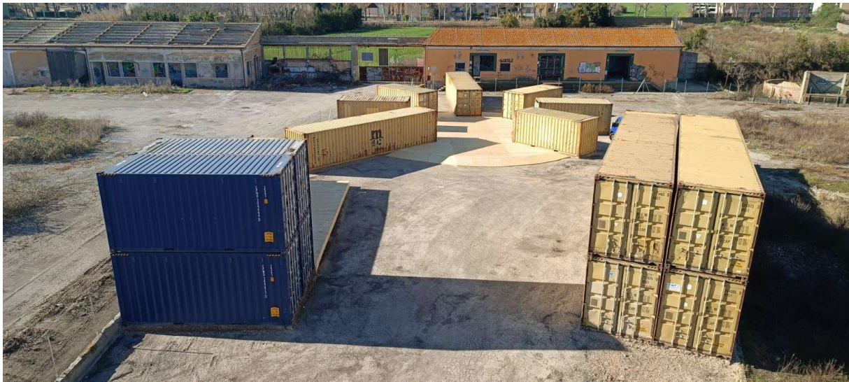
Figure 1 - Air view of the intervention area after the conclusion of the works
