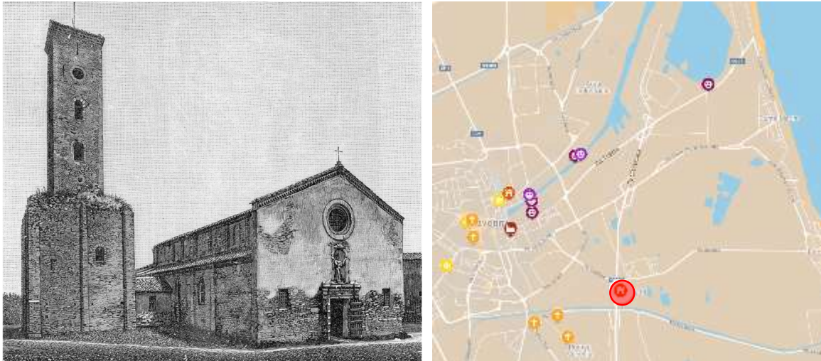
Figure 61. Campanile Chiesa SM Porto Fuori: Historic view and location.
