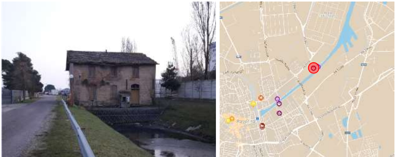
Figure 41. Idrovora Fagiolo: Main view and location.
