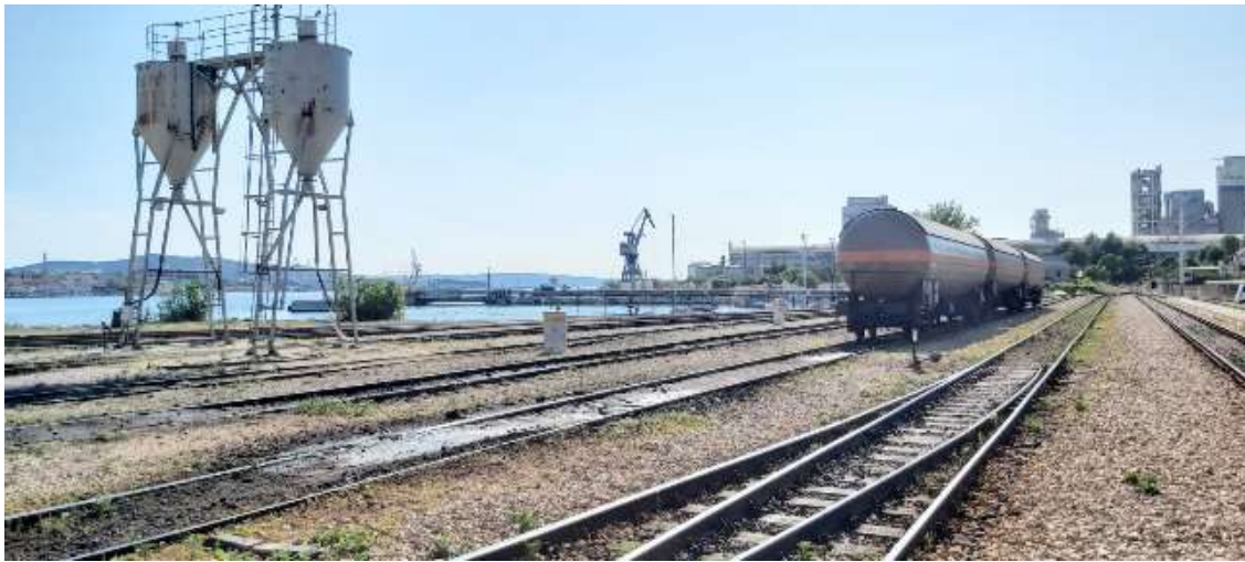
Figure 30. INA tanker berth.
