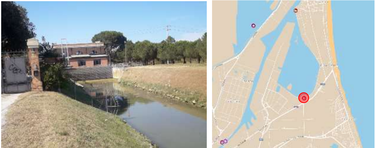
Figure 58. Idrovora San Vitale: Main view and location.
