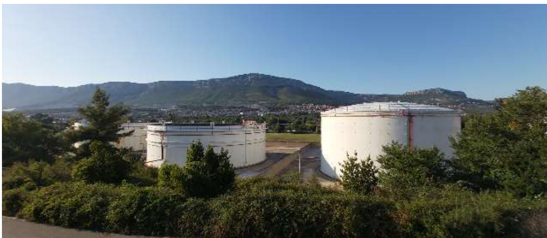
Figure 31. INA fuel tanks.
