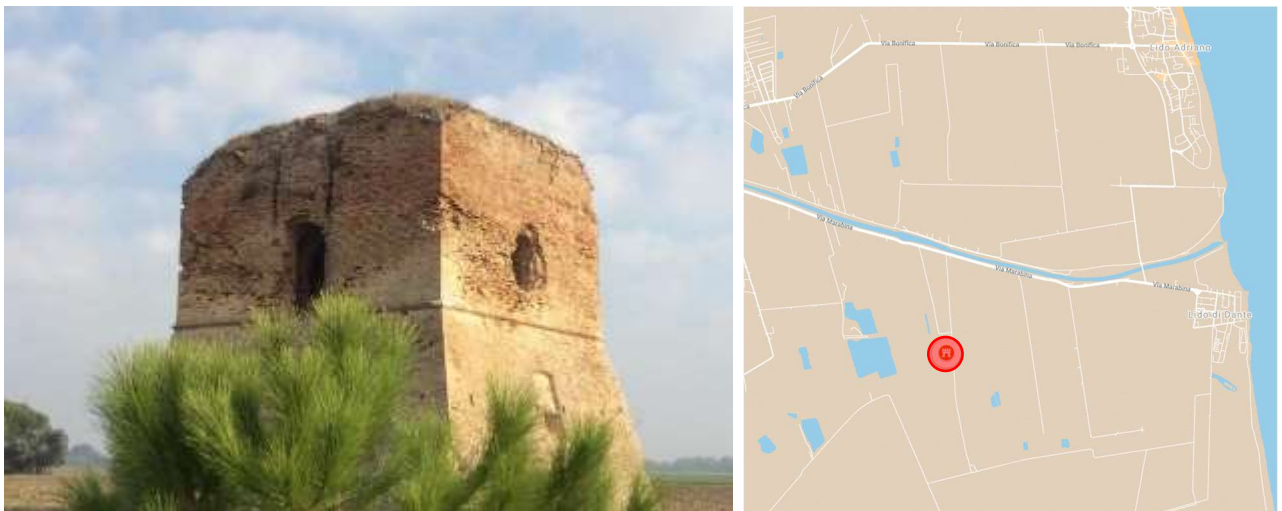
Figure 45. Torraccia: Main view and location.
