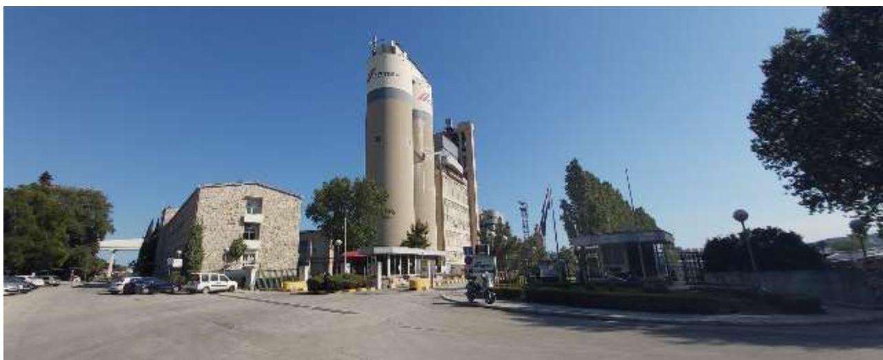
Figure 27. St. Kajo Cement Factory.
