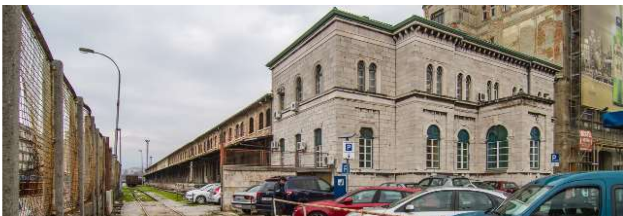
Figure 79. Port Warehouse IIIb.
