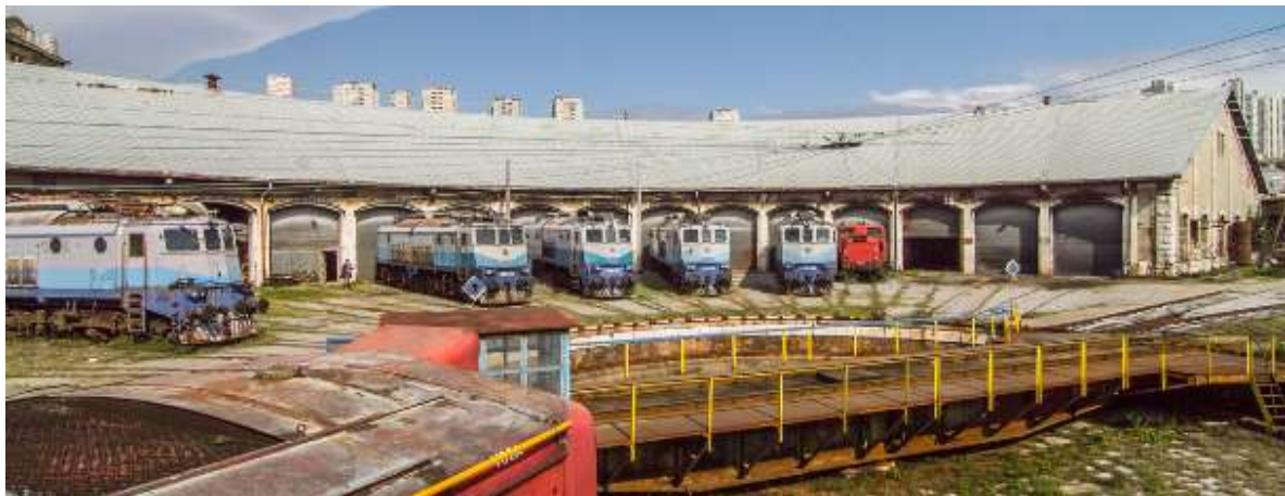
Figure 81. Traction Maintenance Depot.
