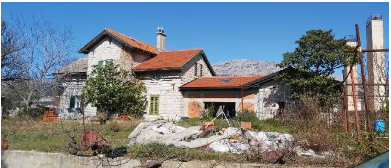
Figure 13. Reception Building at Railway Station Solin.
