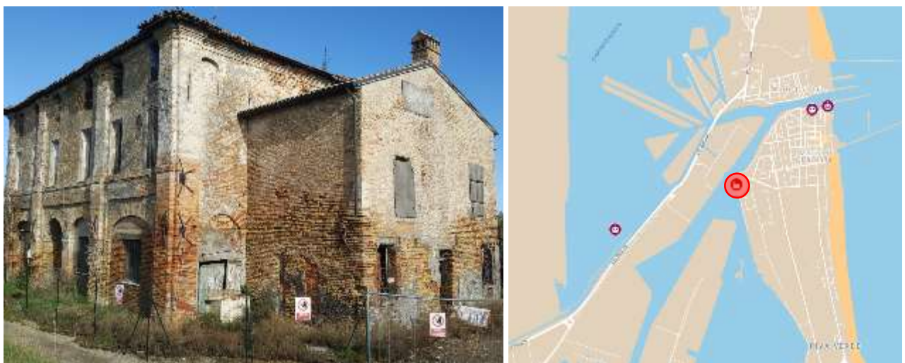
Figure 37. Fabbrica vecchia Ex Marchesato: Main view and location.
