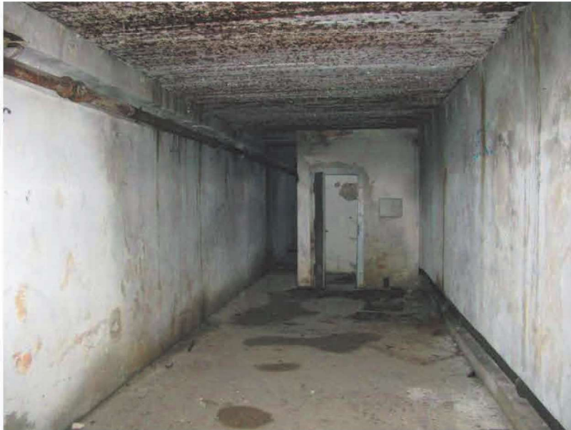
1.7. One of the two main rooms inside of the fort.
