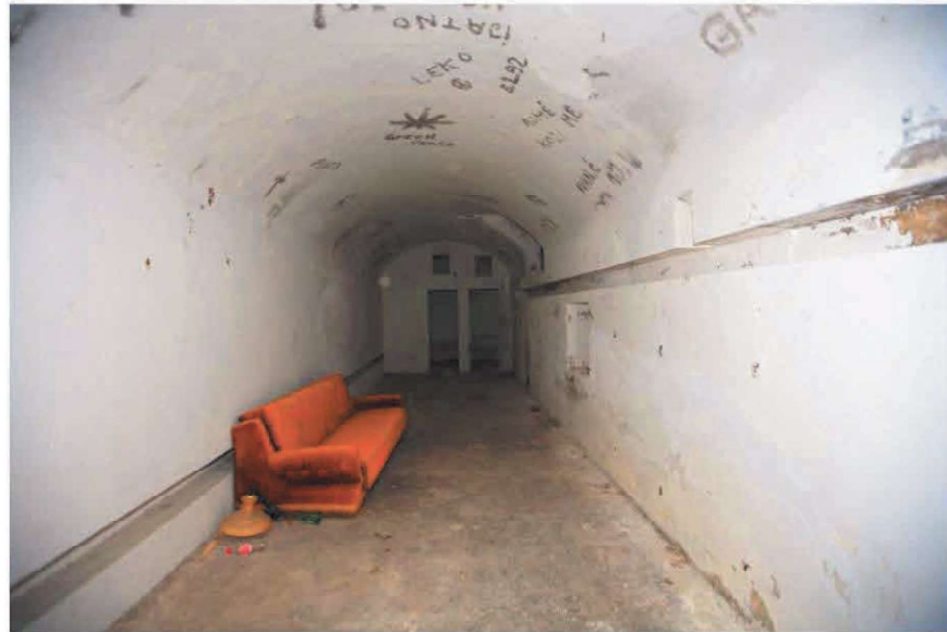
4.3. Internal appearance of the C-30 semiunderground shelter.
