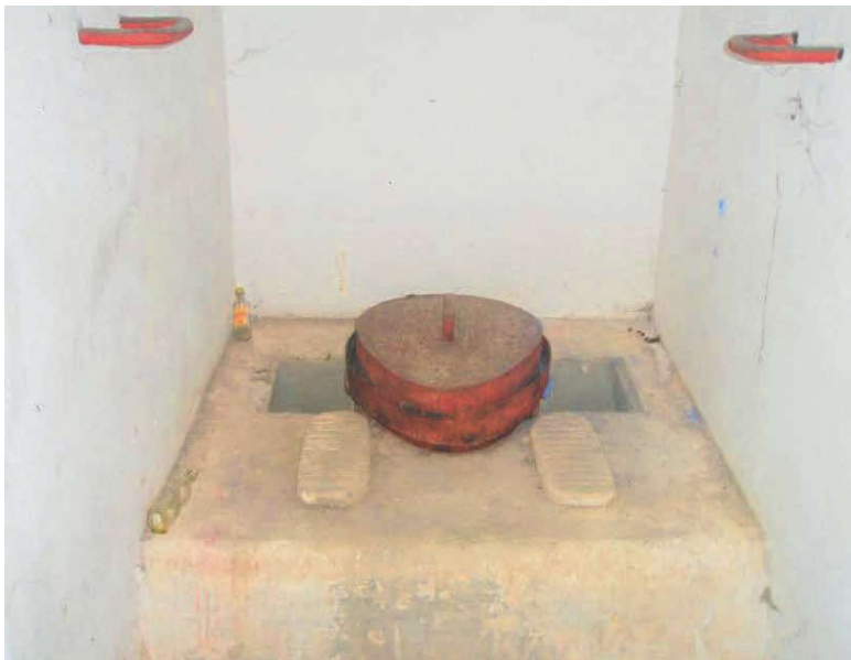
1.8. Well preserved toilets with squat.
