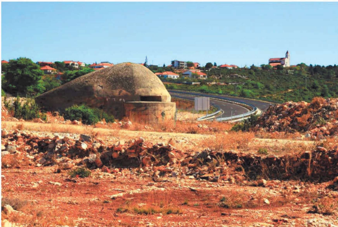
7.2. External appearance of the E-20 bunker.
