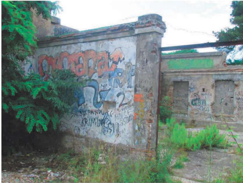
3.5. Entrance to the fort.
