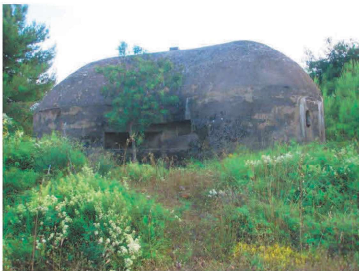
2.5. External appearance of the A-4 marking bunker with combat positions.
