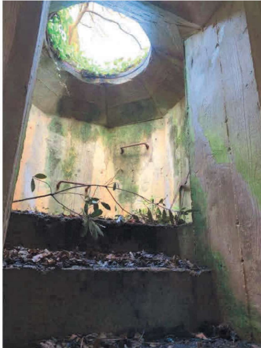
Bunker in front of the entrance of the tunnel.
