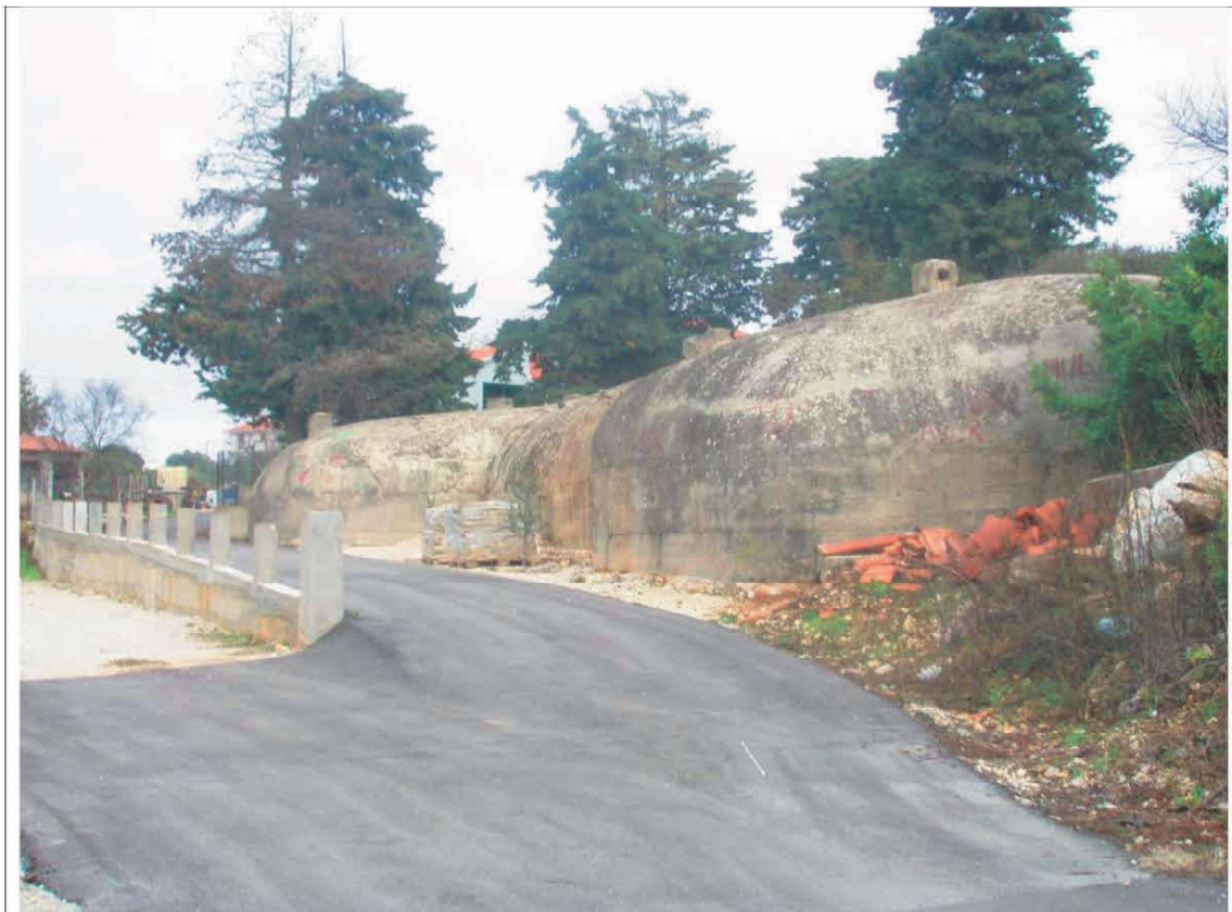
6.3. External appearance of the C-28 semiundergrounded shelter.
