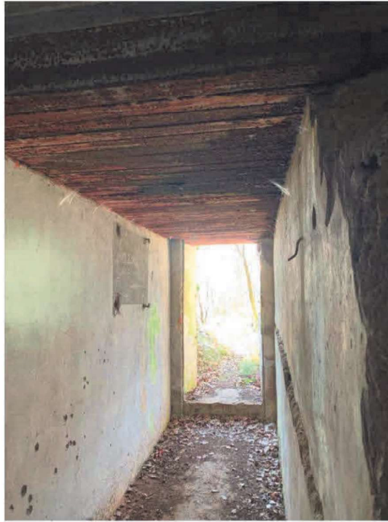
Entrance from the inside
