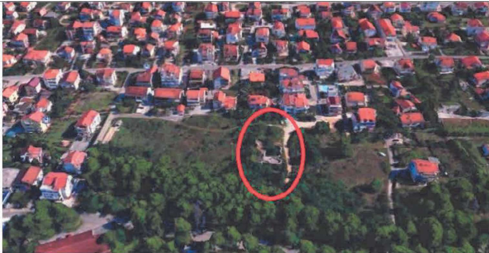
3.3. The position of the fort within the today urban tissue. Source: GoogleEarth
