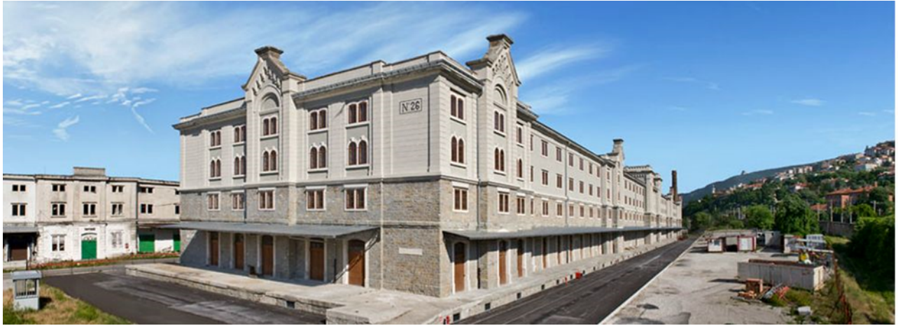
2 – Warehouse no. 26, Old Port
