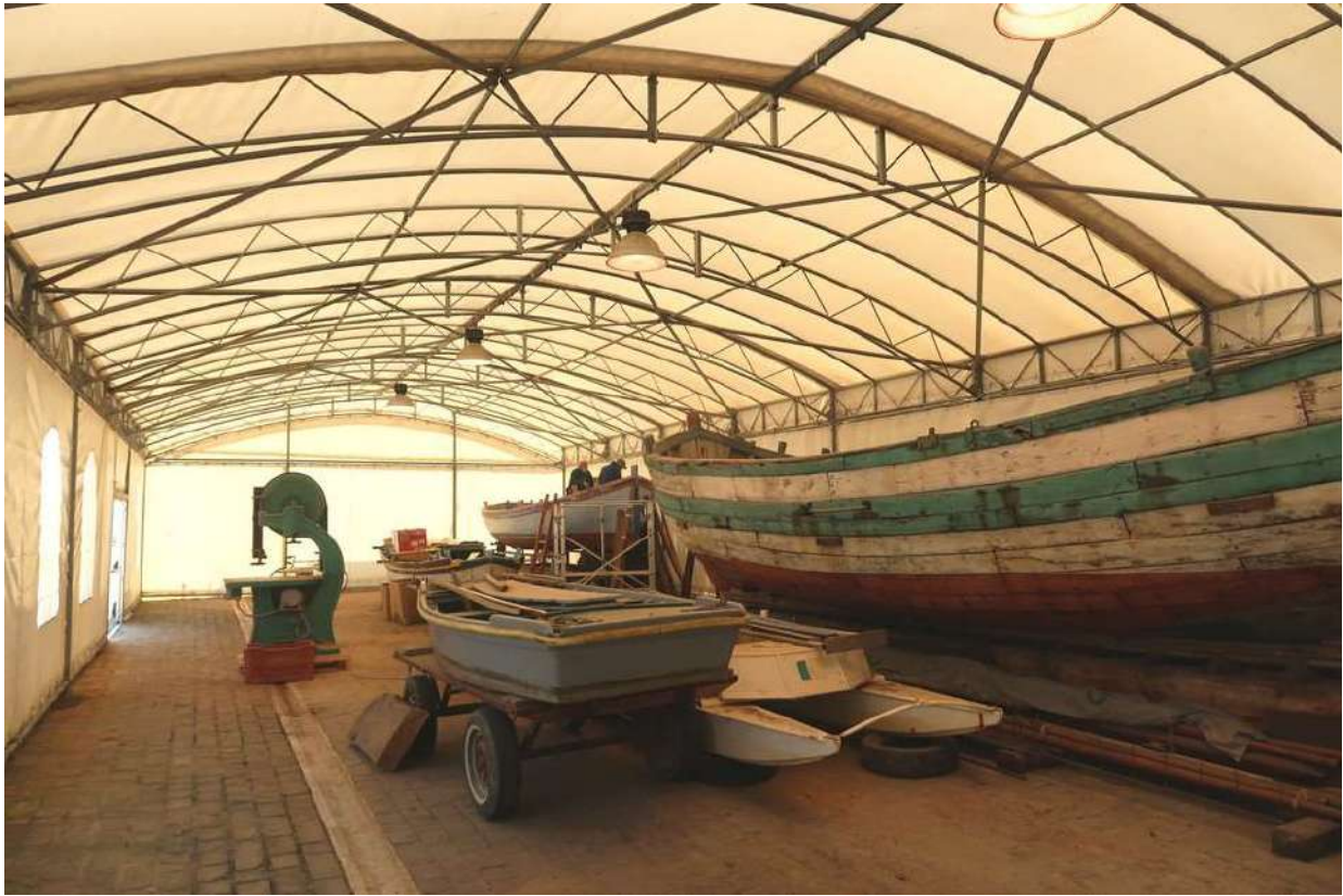
View of the inside of the tensile structure.
