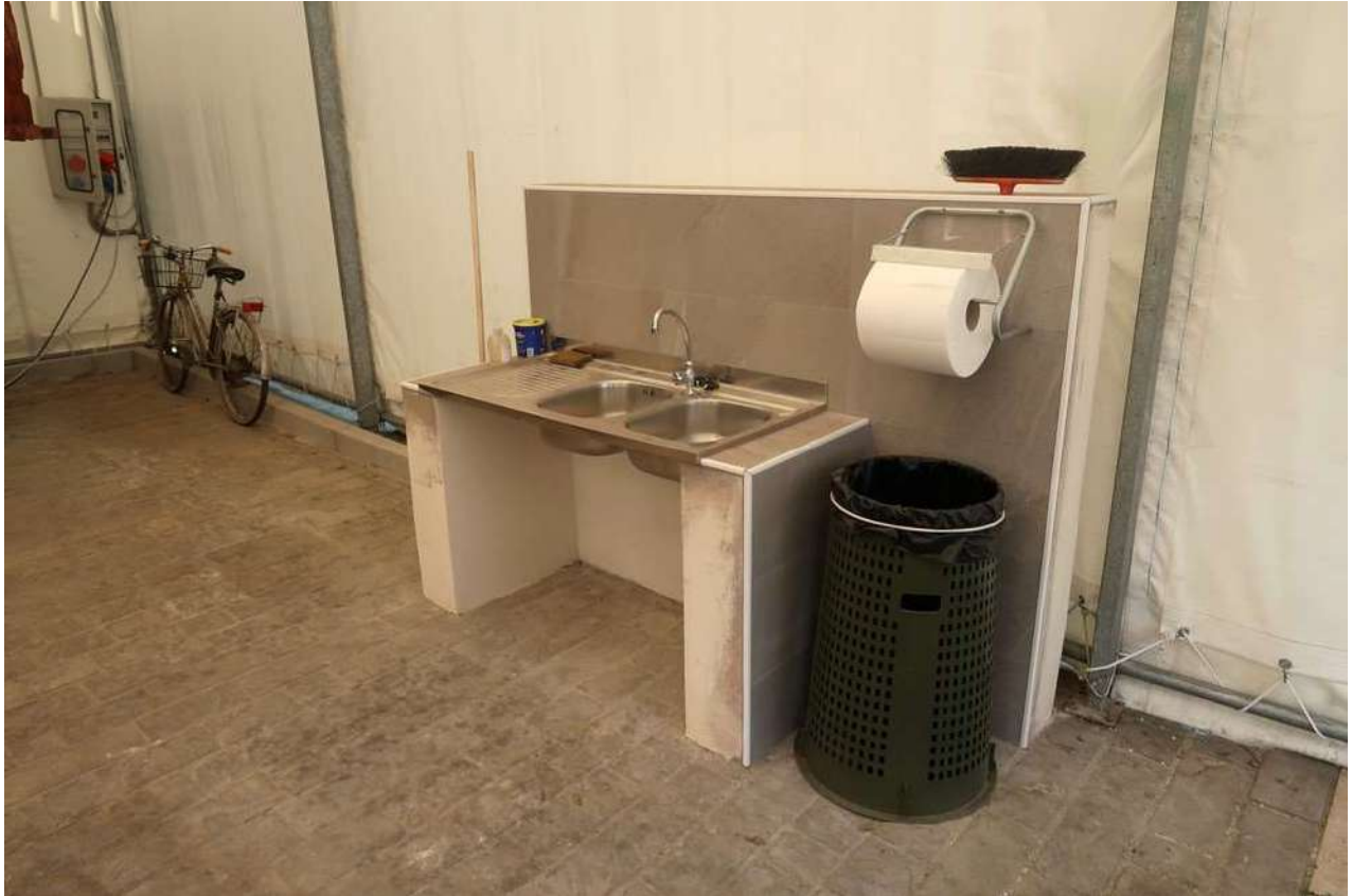
The new plumbing system.
