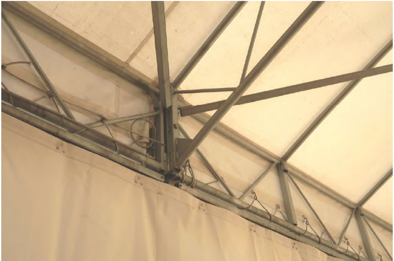
Detail of the support iron elements of the tensile structure.
