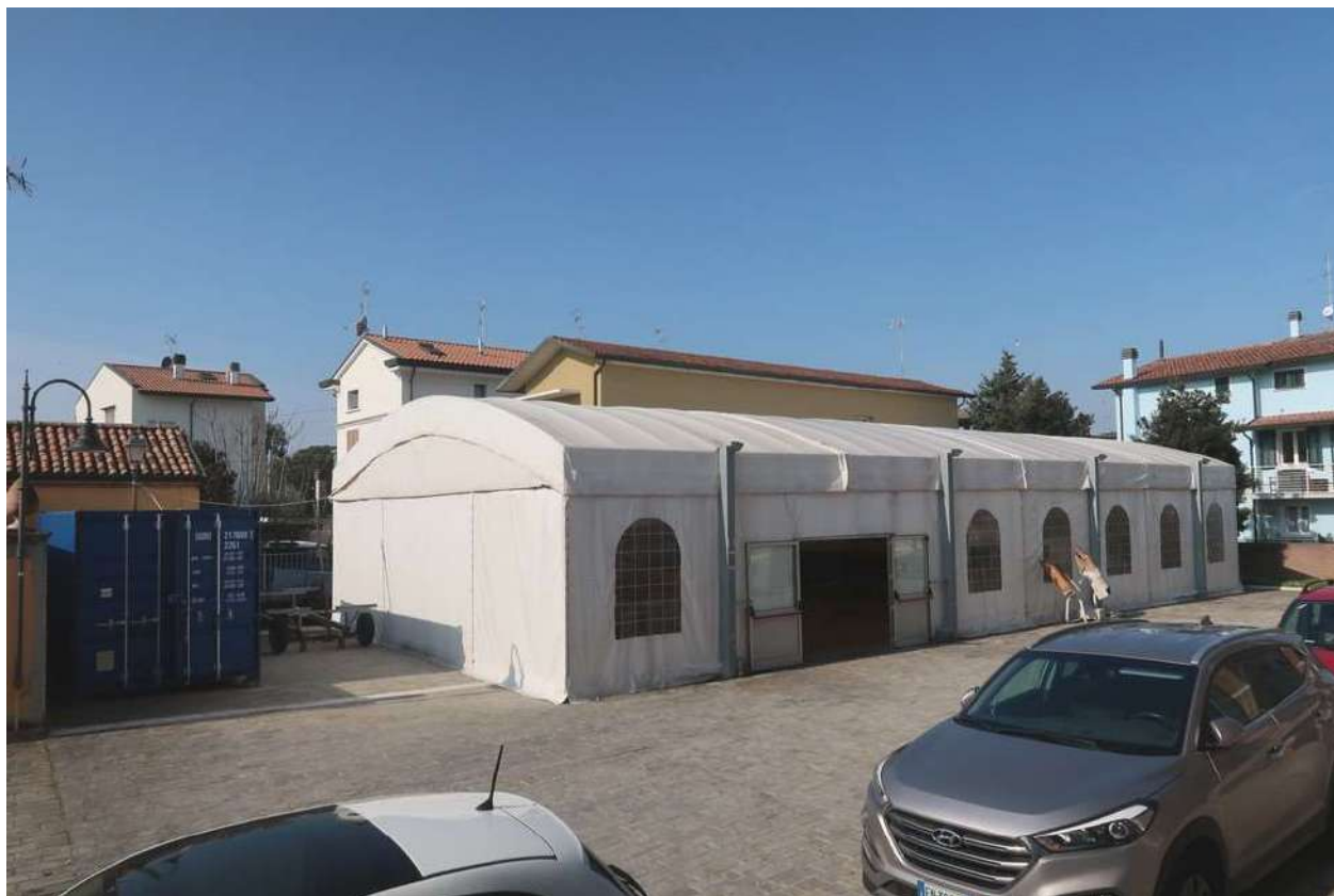
The new tensile structure and the container (on the left).
