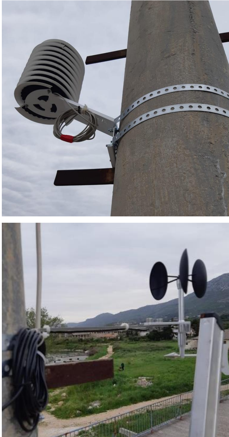
Figure 11. Installation of MeteoHelix and MeteoWind IoT Pro devices
