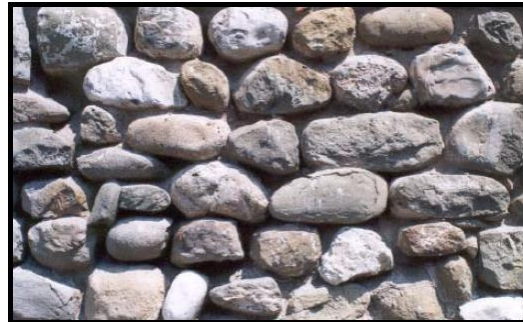
DESCRIPTION: Wall composed of middle size river pebbles roughly worked.
