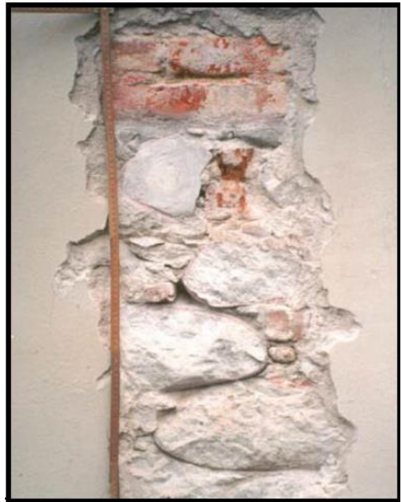
DESCRIPTION: Wall composed of rounded stone with polished surface and with layers of solid bricks.
