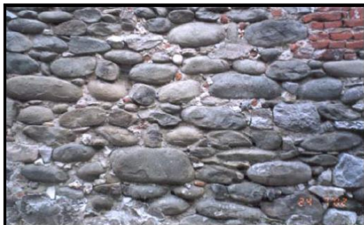
DESCRIPTION: Wall composed of various sizes river pebbles without layers.
