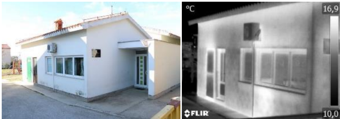
Fig. 23. Kindergarten Franje Tuđmana bb: Structure is brick masonry wall with vertical corner RC confinements, horizontal confinement and RC roof slab covered by roof tiles.
