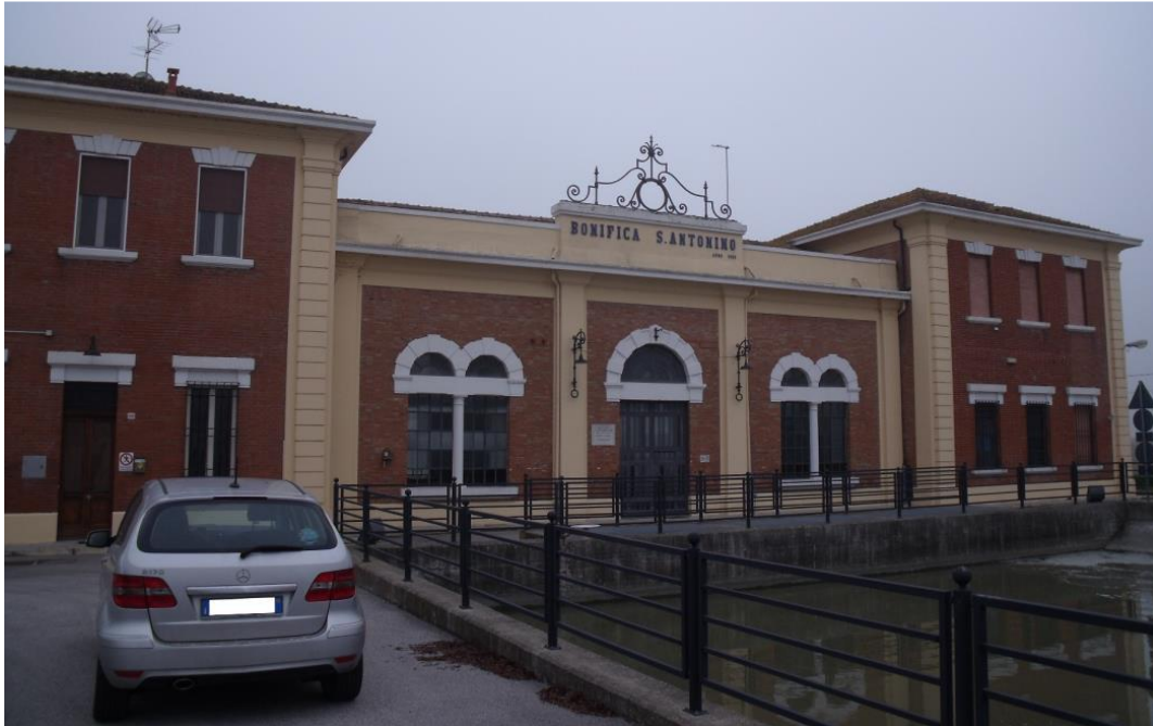
Figure 14. S. Antonino pumping station.
