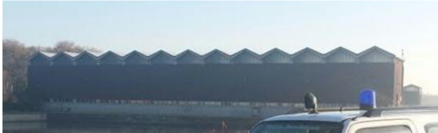
Figure 2. Valle Lepri pumping plant.
