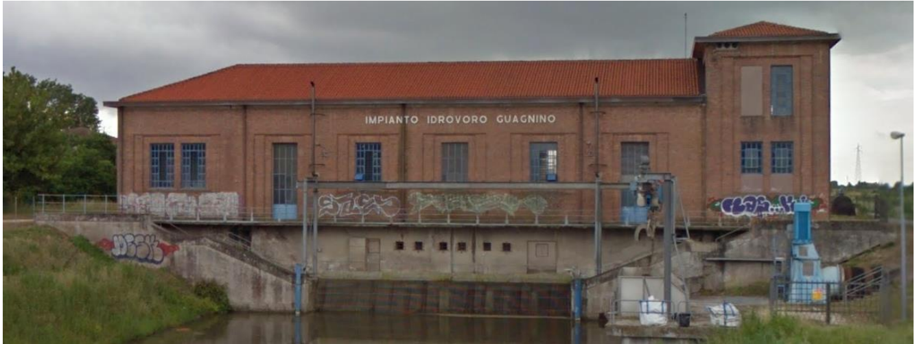
Figure 24. North side of the Guagnino pumping plant.
