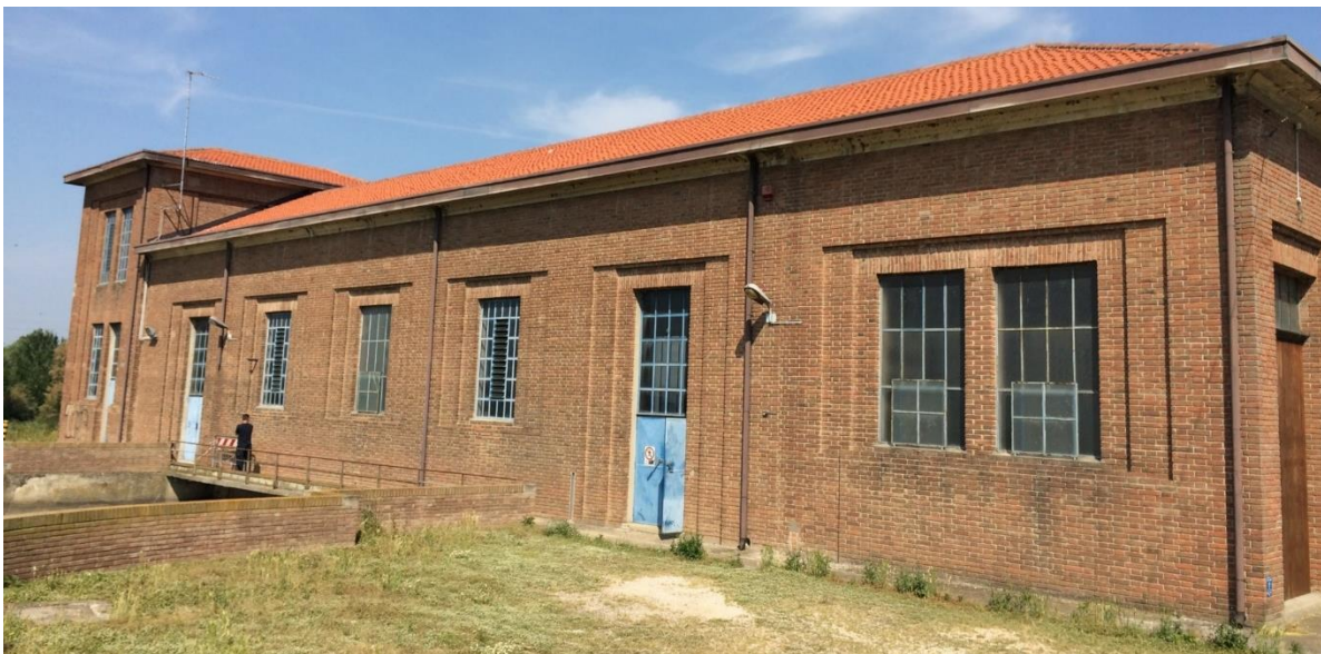
Figura 25. South side of the Guagnino pumping plant.
