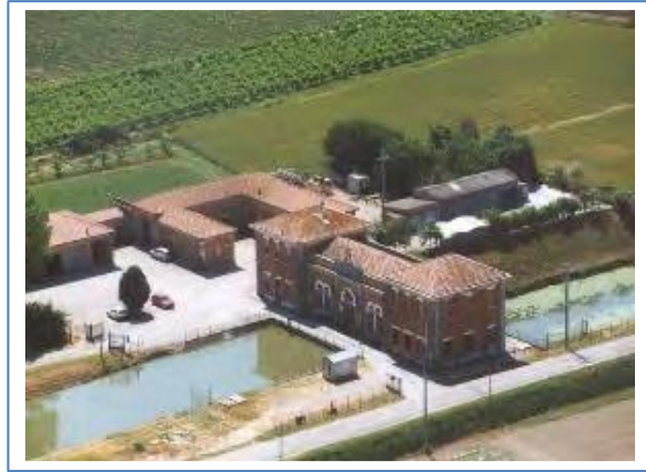
Figure 2., Sant'Antonino old water lifting plant
