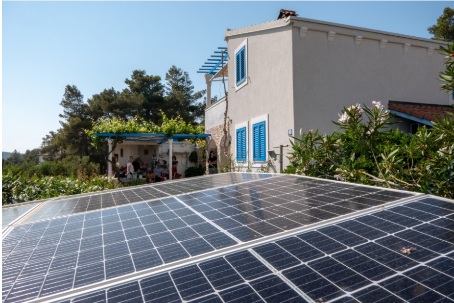
Study visit - solar photovoltaic panel serving as garage rooftop in Vela Luka
