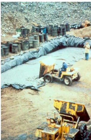
Picture 6: Improved pit near a recovery site on shore
