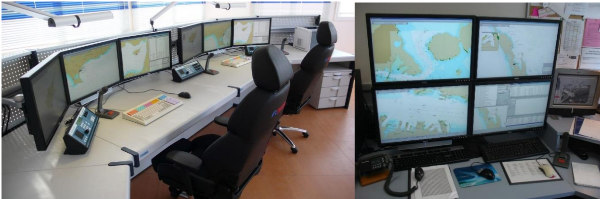
Figure I-4. Example of an operations center
