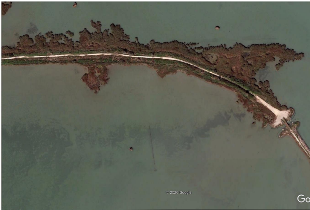
Figura 4-5 Detail of the north embankment and the gate
