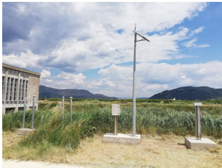
Figure 18 Monitoring location GW_MON_P4 and GW_MON_D4
