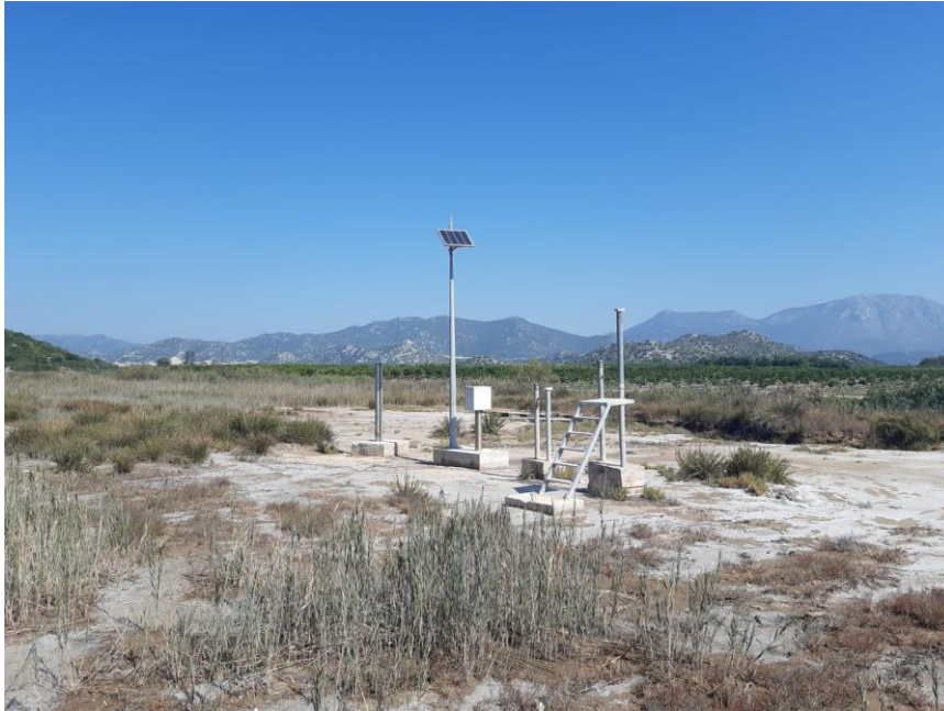
Figure 13 Monitoring location GW_MON_P1 and GW_MON_D1
