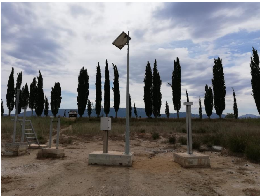
Figure 12 Monitoring location GW_MON_P1 and GW_MON_D1
