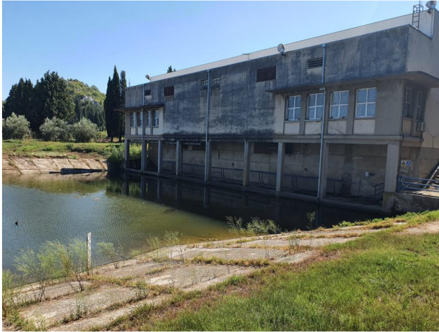
Figure 19 Monitoring location SW_MON_1
