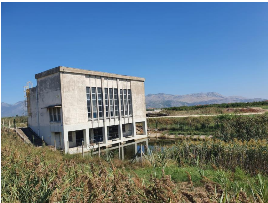
Figure 24 Monitoring location SW_MON_3
