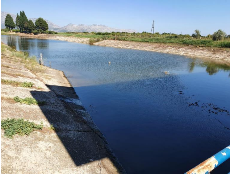
Figure 21 Monitoring location SW_MON_1
