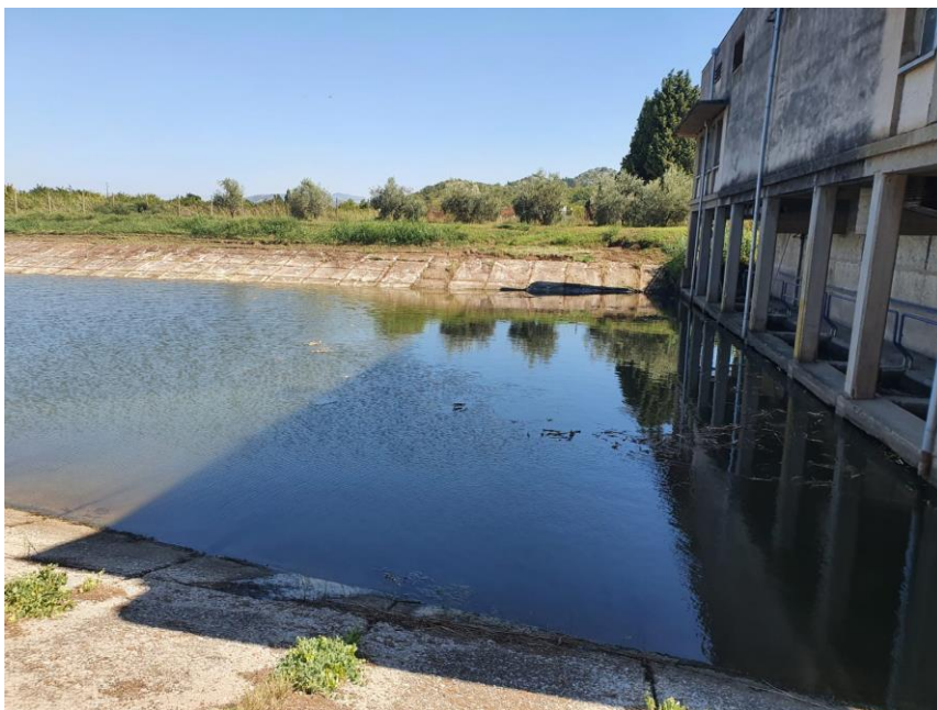
Figure 20 Monitoring location SW_MON_1
