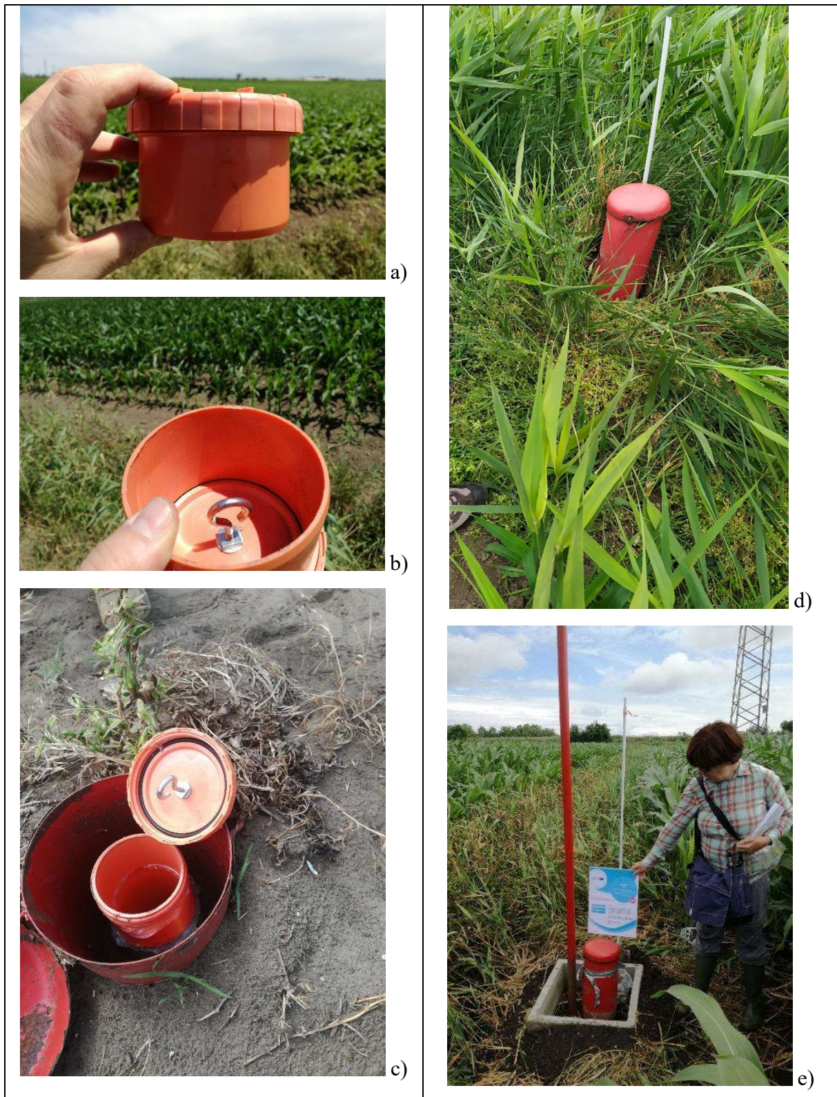
Fig. 7– a-c) Detail of the screw top with ring used to fix the cable of the sensors; example of protection measures adopted to avoid SI piezometer damage during the farmland works: d) previous inadequate method with simple thin white pipe, e) new steel pole red-colored, and concrete square manhole.
