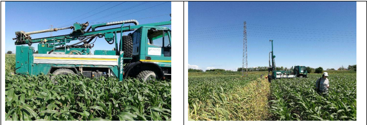
Fig. 8 – Drilling machine used for the installation of the new MoST piezometers.
