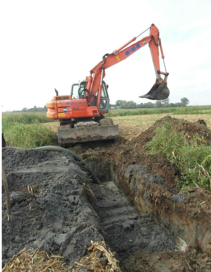
Fig. 3 – Excavation of the trench and positioning of the pipe.
