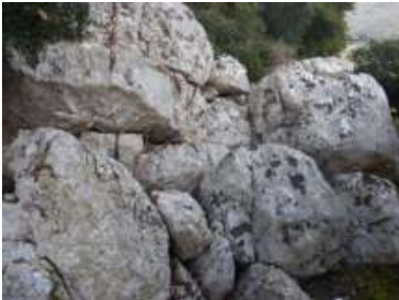
Figure 6.22 Fractured massive limestones, Veliki obalac
