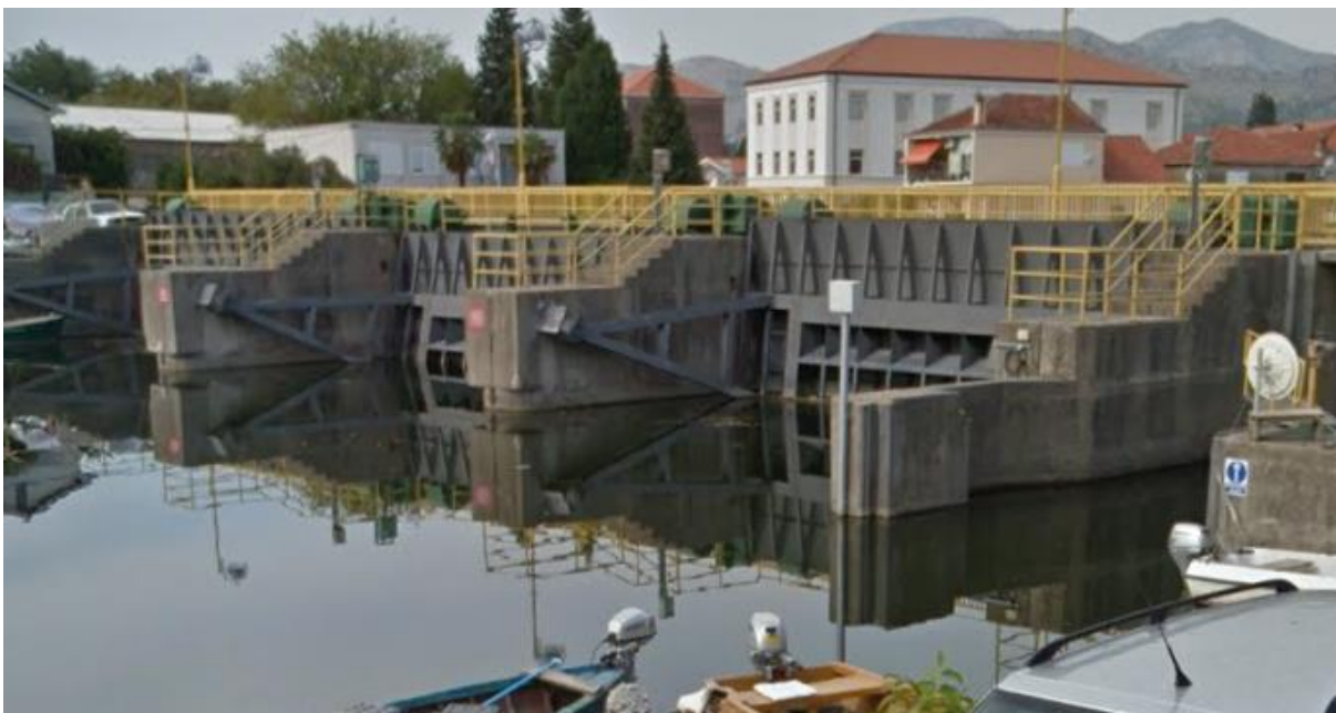
Figure 8 The OU river gates (Google Street View)
