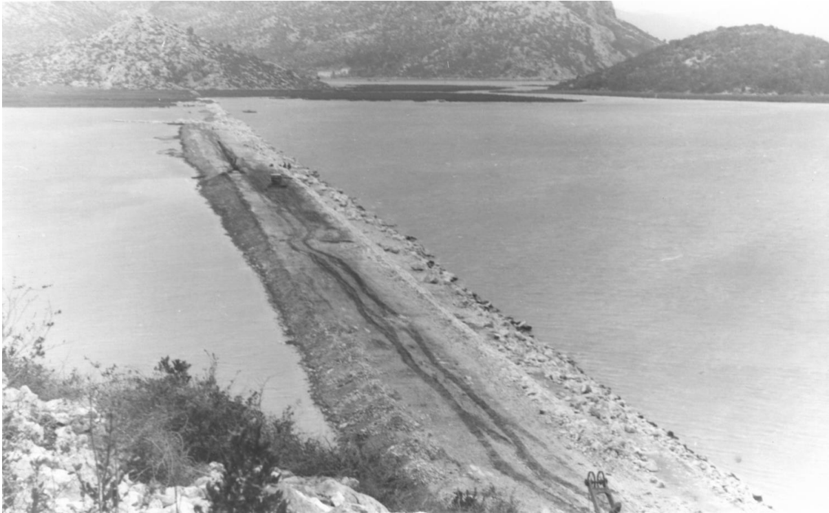
Figure 7 Diga construction sand refill (mid of 20th century) - view from the Galićak hill
