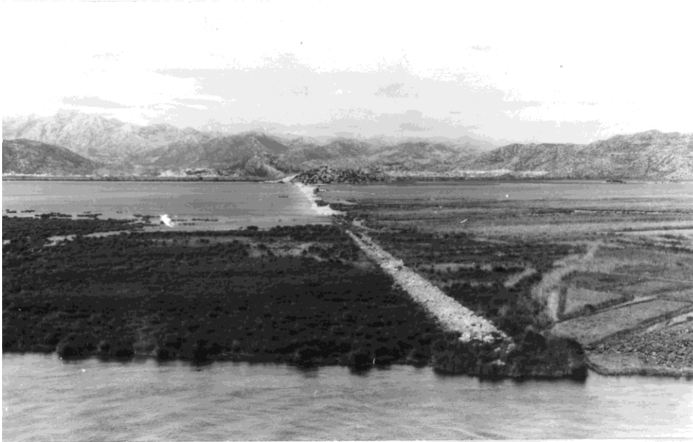
Figure 5 Diga construction (mid of 20th century) - view from the Mala Neretva
