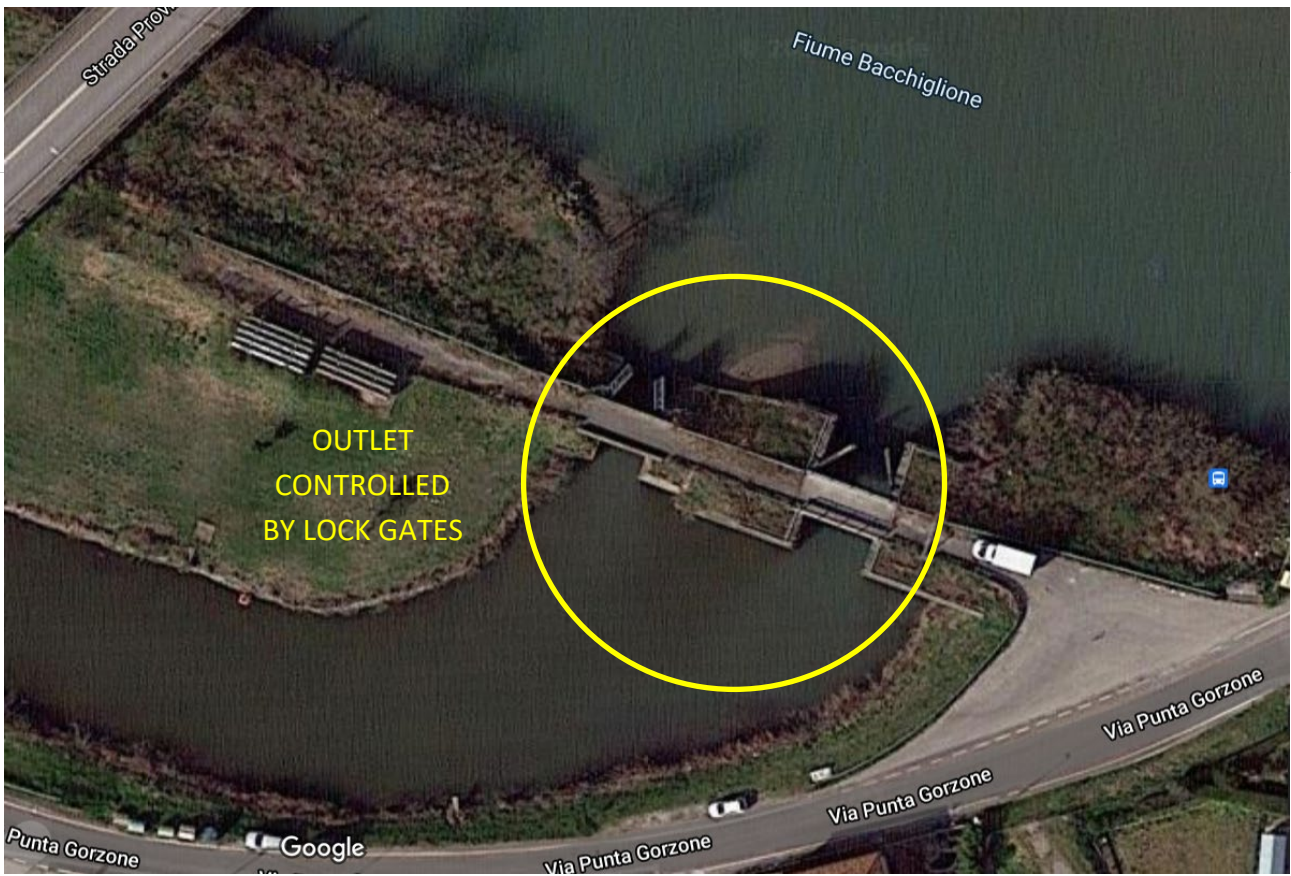
Figure 7 - Canal Morto outlet controlled by lock gates
