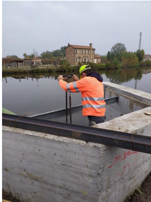
Fig. 18 - Worker opening the valve at the water catchment of the pipe.
