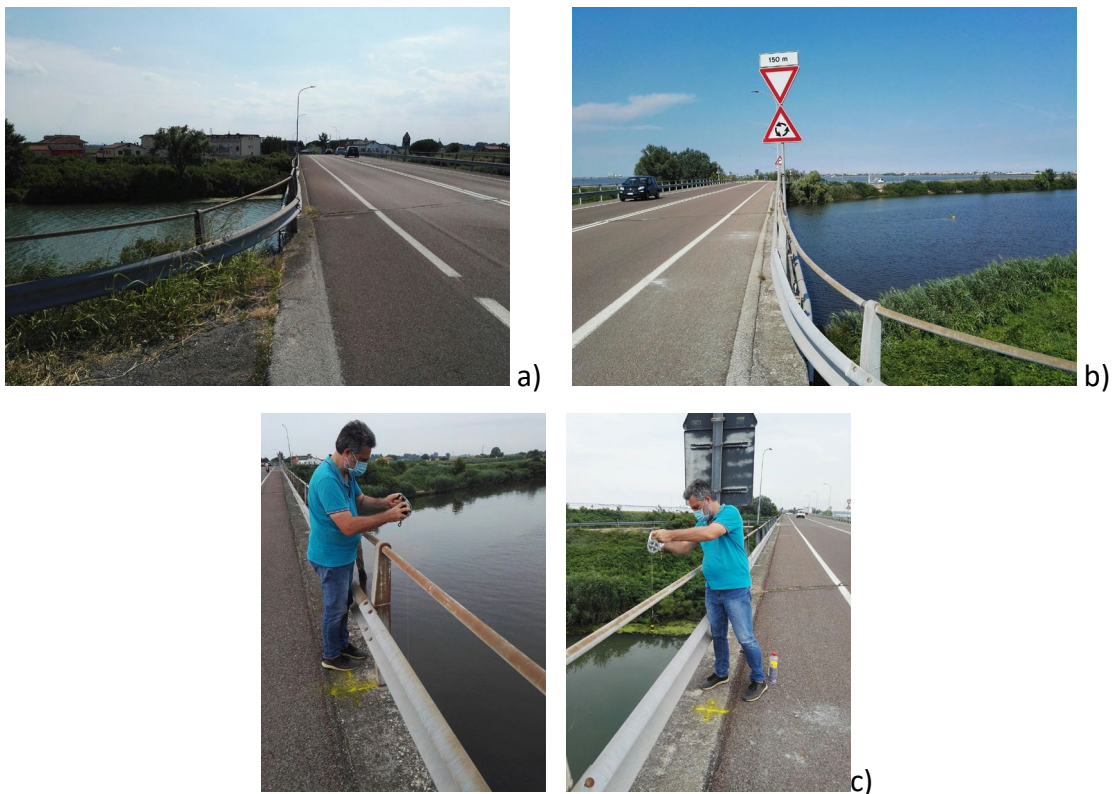
Fig. 6 - Monitoring at Ca' Pasqua bridge.
