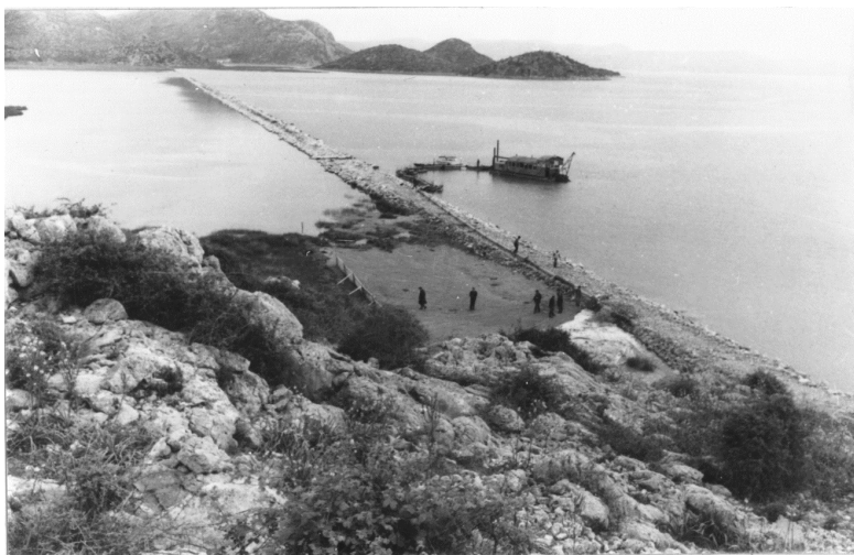
FIGURE 1. COASTAL EMBANKMENT DIGA DURING CONSTRUCTION
